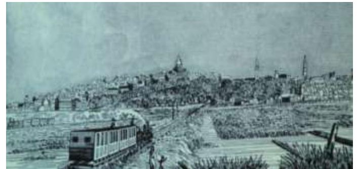
Railroads crossing the basins created problems
