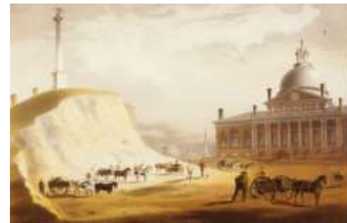
Filling the Mill Pond
