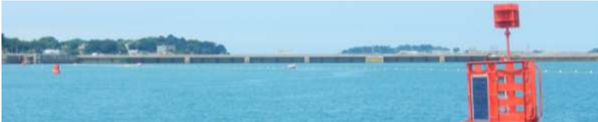
A wide-angle view of the upstream side of the dam.
