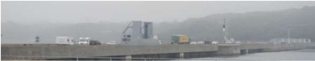
A closer view of the upstream side of the dam.
