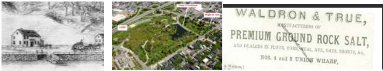
PORTLAND (Top) [L] 1845 map shows original extent of mill pond. [C] By 1852 a railroad crossed the pond and filling of Baco Cove decreased available water for milling. [Bottom] 1842 pencil sketch of the mill on the dam. [C] Modern aerial shot shows what’s left of the pond. The red star shows site of the mill, now covered by a city street. [R] Advertisement of City Mills, one co-owned by George W. True.
