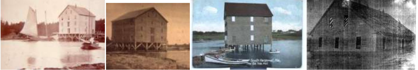
Four views of the mill at Basin Cove in Harpswell.
